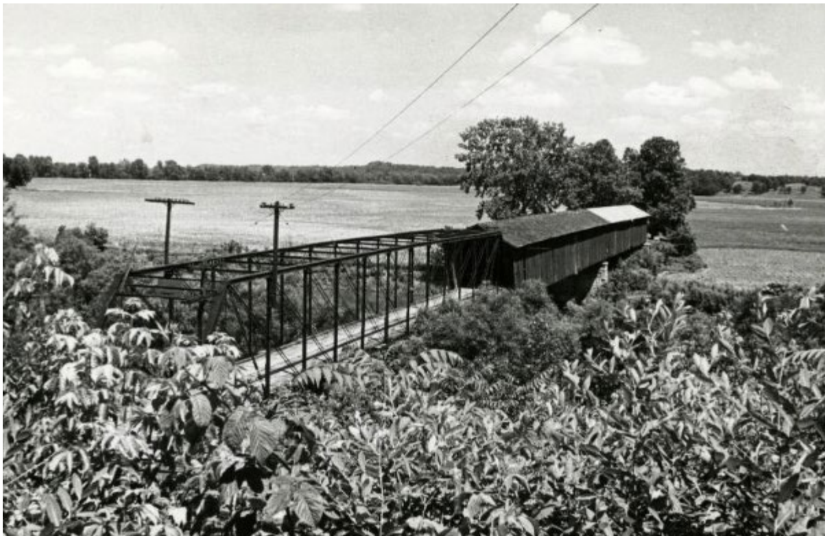
Gosport Covered Bridge, 1941 (Indiana Historical Society, M0836)
