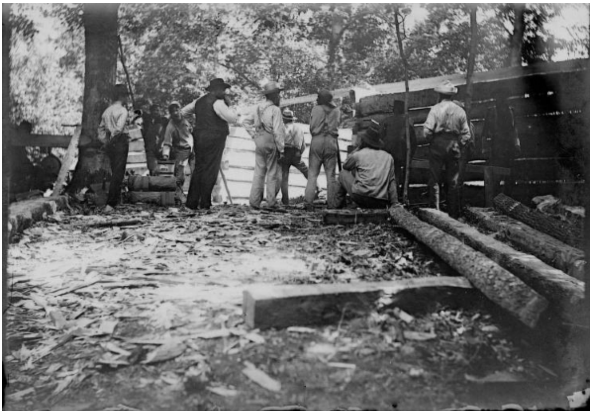
Log Cabin Under Construction, Woollen's Garden, ca. 1910 (Gift of Samuel E. Perkins, IV, Indiana Historical Society)
