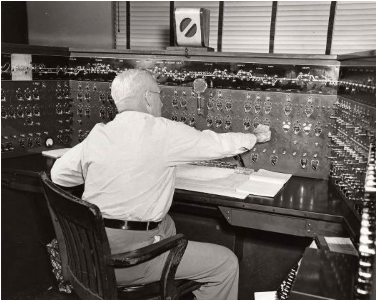
Nickel Plate Railroad Switchboard Controller, ca. 1940 (Richard Simons/ Indianapolis Star Magazine , Indiana Historical Society )
