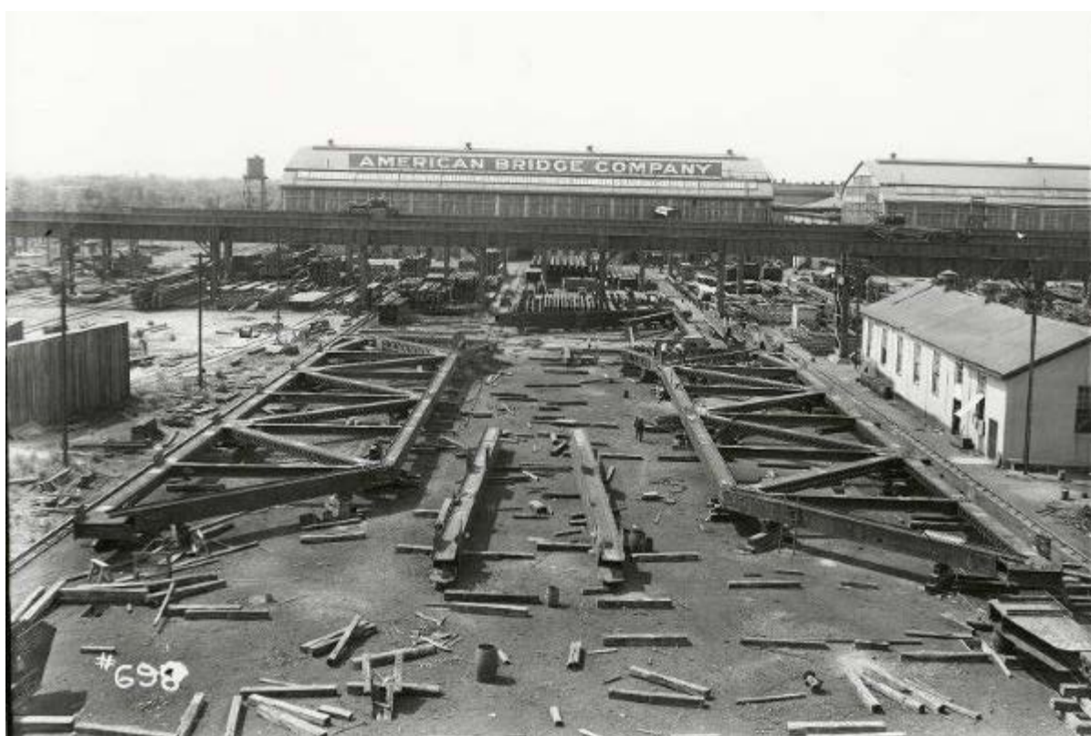
Bridge Trusses in Yard of Gary American Bridge Company Plant, ca. 1918 (Indiana Historical Society, P0349)
