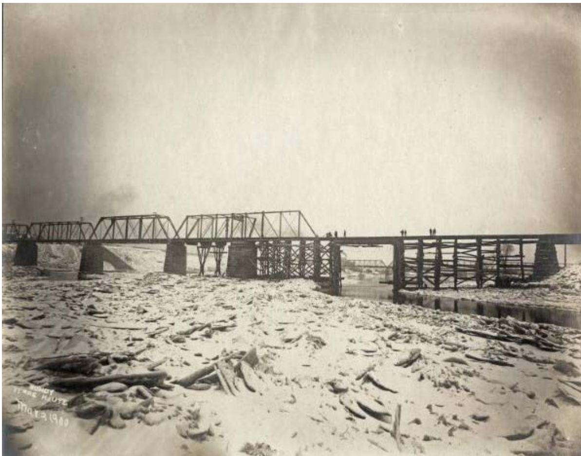
Big Four Railroad Bridge Reconstruction, 1900 (Indiana Historical Society, P0333)
