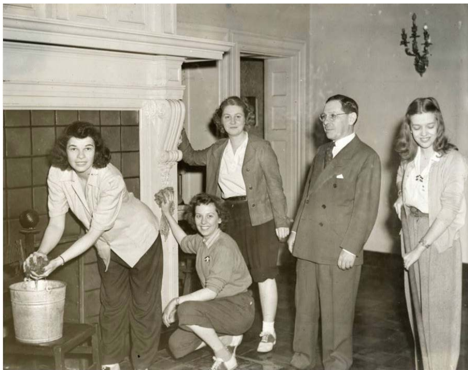
Cleaning at the Maennerchor Building. (Indiana Historical Society)
