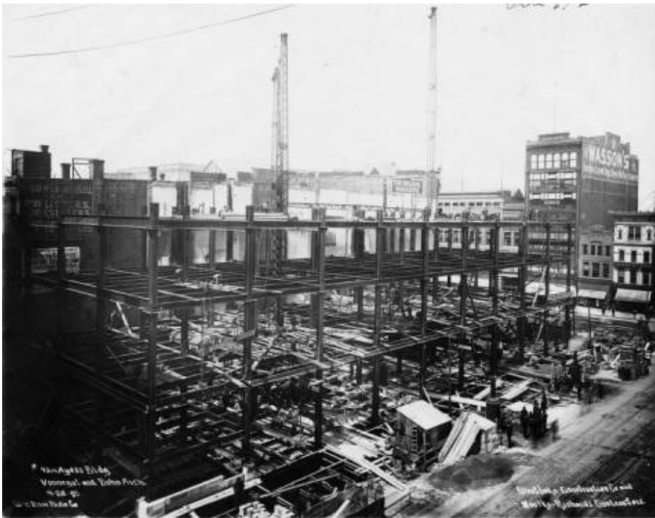
Ayers Building Construction (Bass Photo Co. Collection, Indiana Historical Society)
