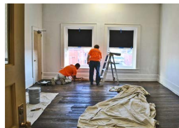
Painting and plaster repair completed before the new cabinets are installed.
