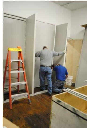
Installing the new garment storage units.
